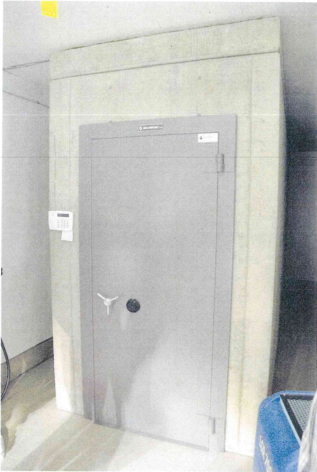
Photograph of a vault being used at a small MMPR licensed producer facility. Multiple secure doors and areas monitored by video surveillance have to be passed to get to this area.
