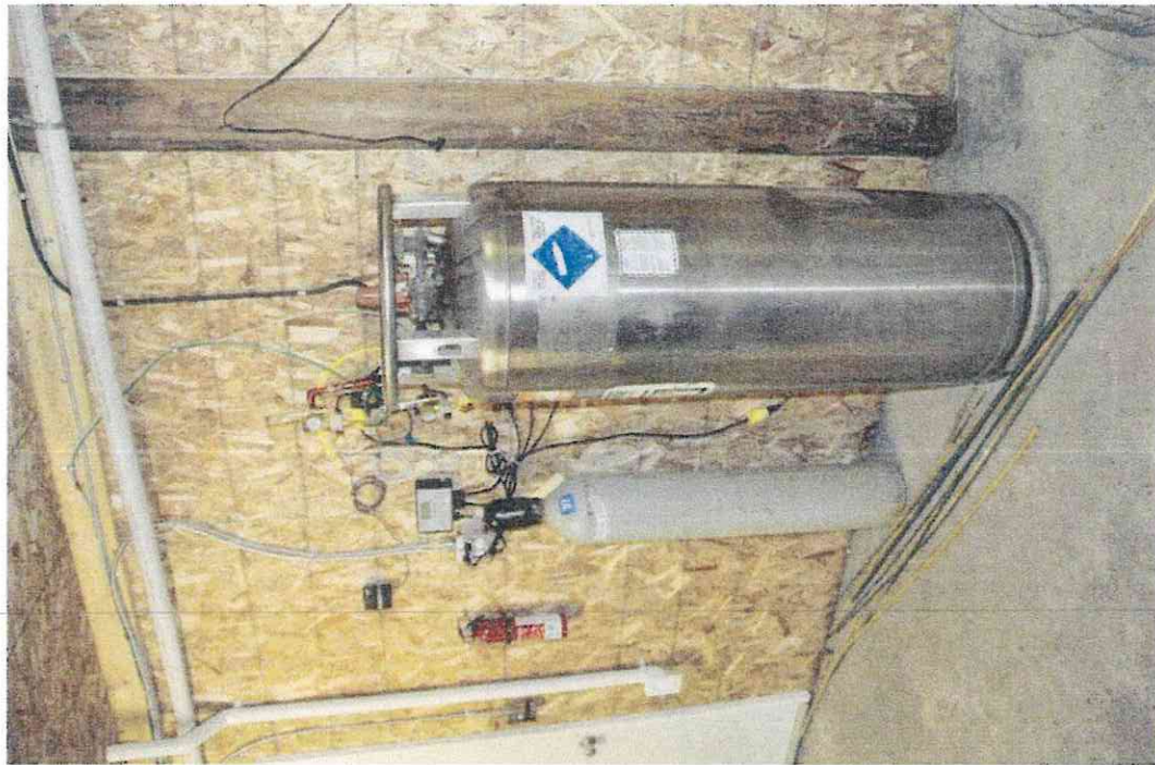
These commercial size CO2 tanks were located at a MMAR production site. Inadequate monitoring and leak testing could result in the exposure of fatal doses of CO2.
