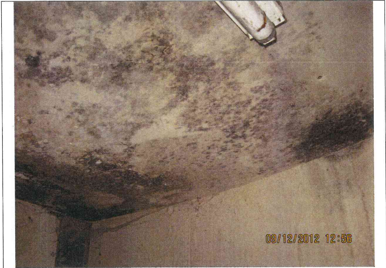
Photo 3 Example of: Major Mould Growth (2) Description: This photo shows an example of major mould growth (dark and spotted staining throughout drywall). Major mould growth is to be considered > 1m^3 .
