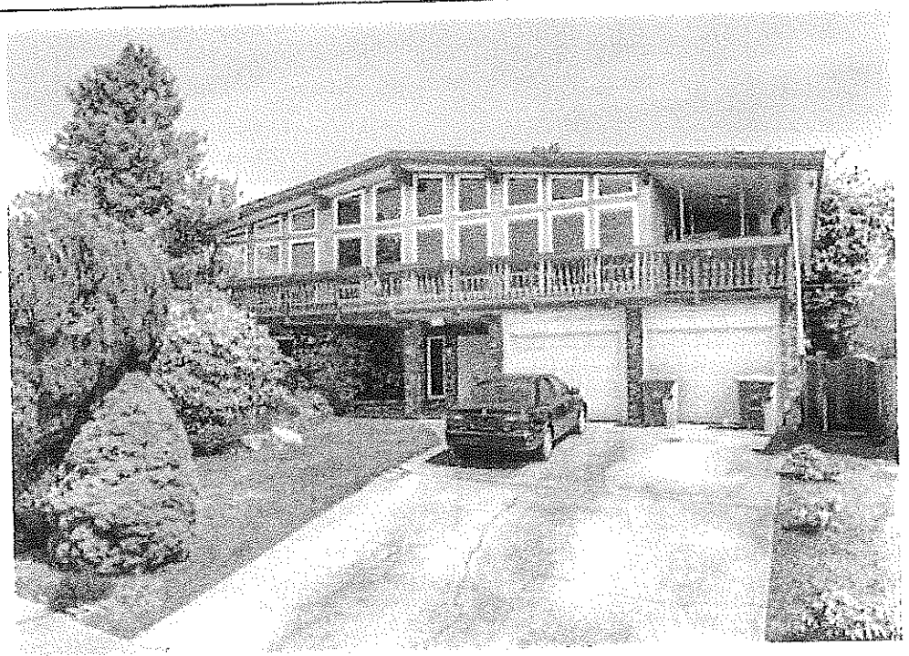
Subject Building No. 3
