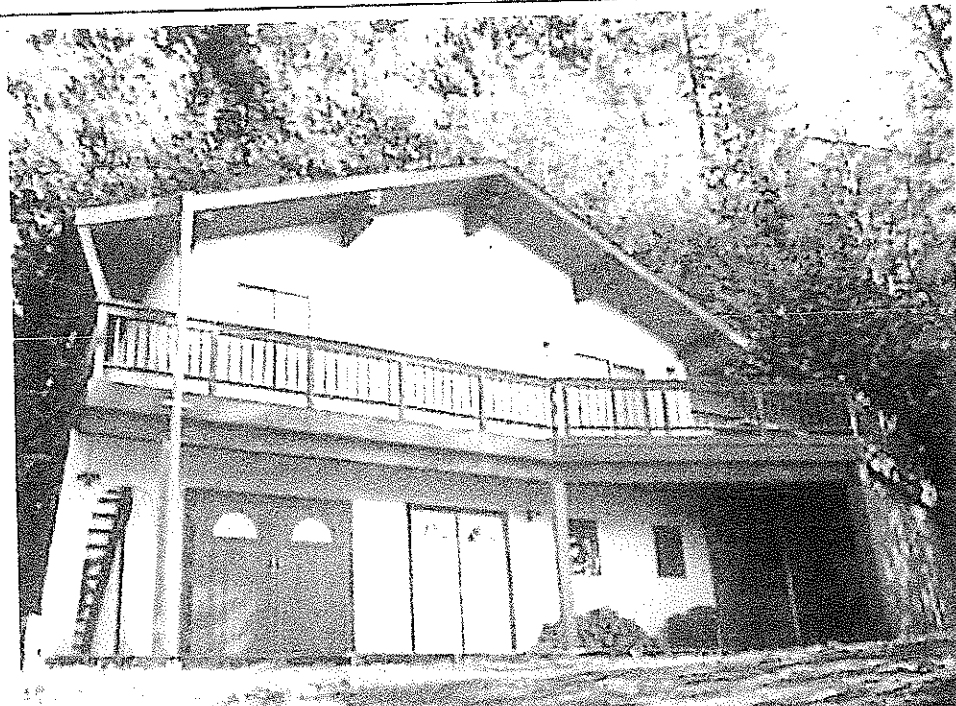
Subject Building No. 1
