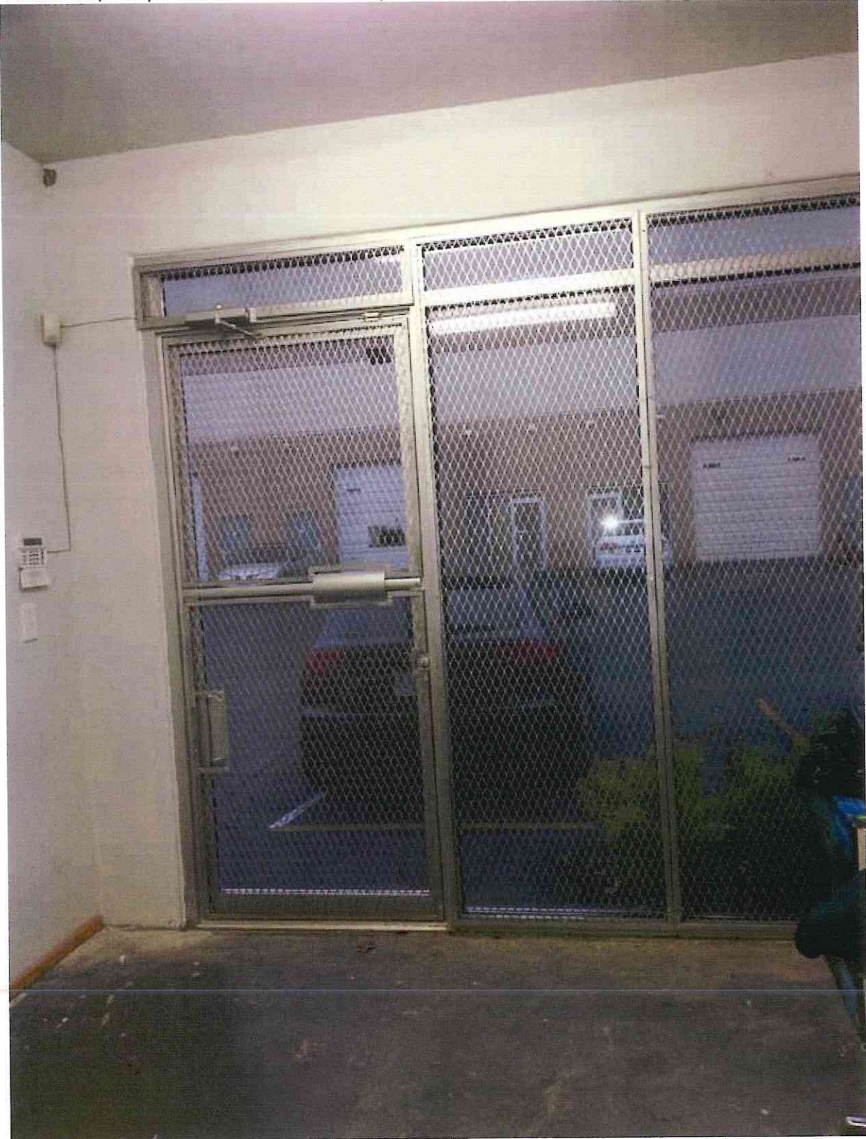
Front Office / Entry: Secured with Steel Security Mesh
